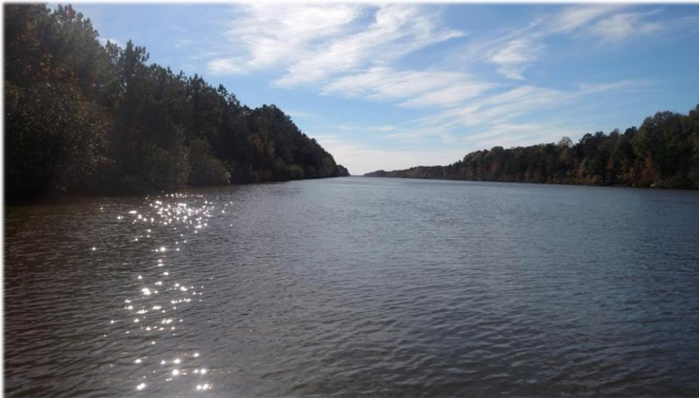
**Left:** The Tennessee-Tombigbee Waterway (TTW) was completed in 1984 and is owned by the U.S. Army Corps of Engineers. It is still the largest earth moving project in U.S. history. The navigation channel throughout the TTW is 300 feet wide and a minimum of 9 feet deep.
